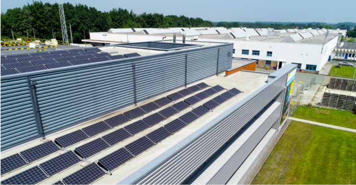
BUILDING OF THE NEW TECHNICAL CENTRE IN STRÉPY-BRACQUEGNIES
